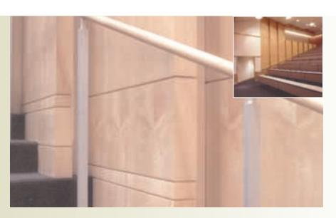
"The most challenging piece of architectural woodwork in the project was creating the complex configuration and geometry of the 'saw-tooth' side wall panels while working with the floor and ceiling profile. The design goals of creating a beautiful and inviting space were achieved in this project."
