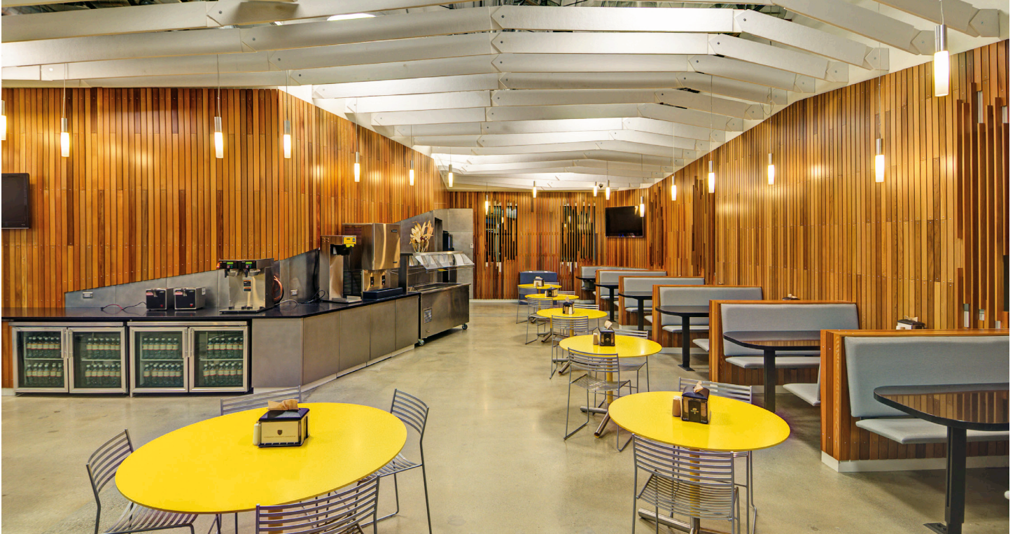
Our scope of work in the Café area included the banquette seating with granite tops and bases, stainless steel wall paneling, stainless steel cladding on the base cabinets along with the cedar paneling and ceiling baffles.
