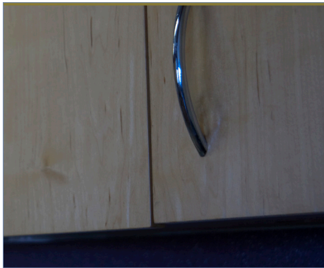
Euro hinges can work their way out of adjustment.
