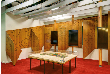
Kiosk Area — \frac{3}{4} " Bamboo with random holes throughout. Kiosk monitors are hung from 2x6 Douglas Fir posts.
