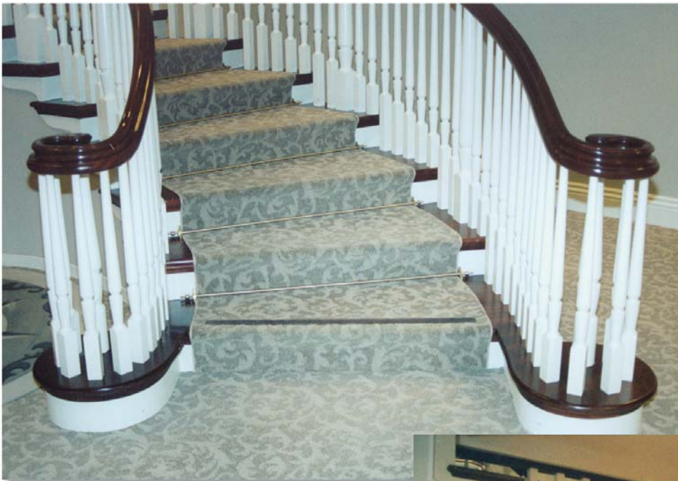
The volutes at the start of this stair fulfill the ADA handrail requirements by extending in front of the starting step.
