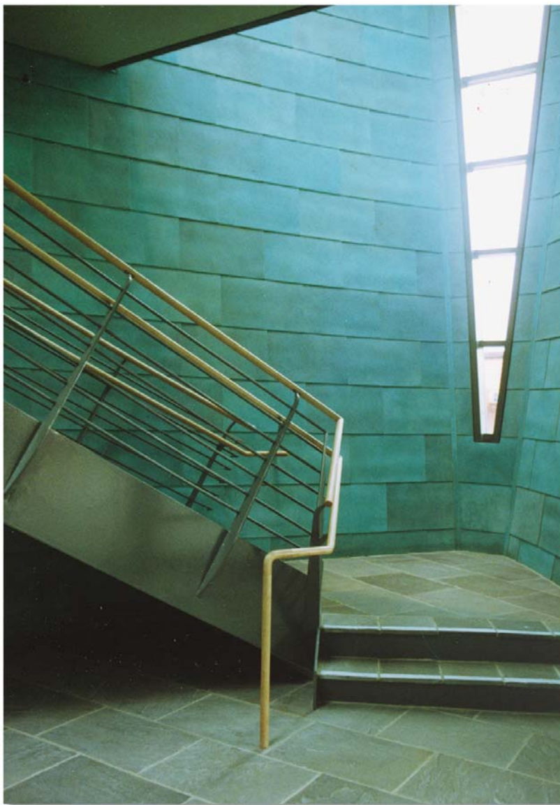
This starting treatment required a 1/2 x 3/4-inch steel bar inside the wood rail from the floor to the first handrail bracket.
